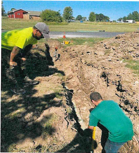
Repair sewer line break on Optimus Dr.
